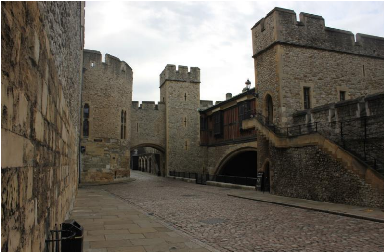
Figure 3 - Wakefield Tower (Left) and St Thomas's Tower (Right)
